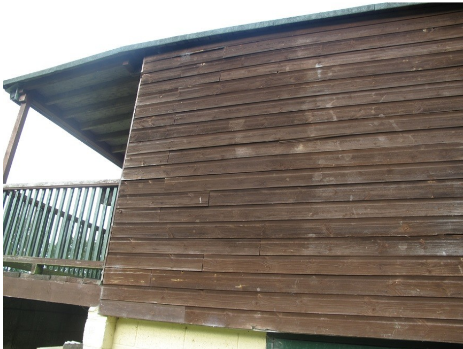
Fig 5 Note the timber frame sitting on breeze blocks with timber cladding.
